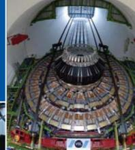
The large pieces of CMS, weighing between 200 and 2000 tonnes each, are lowered 100 m into the cavern before being assembled into position.
